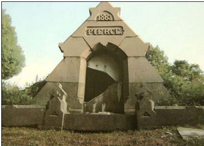
The vandalized crypt at the Old Hill Burying Ground in Newburyport.
